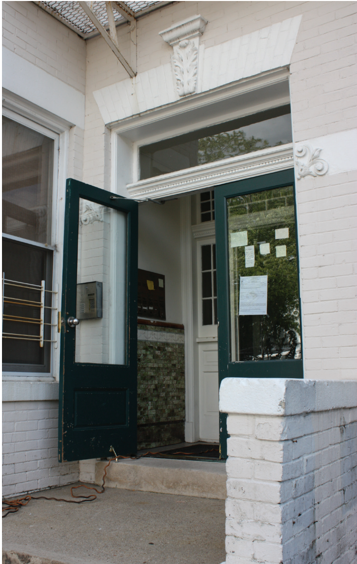
[11] A vestibule helps retain interior conditioned air in the living space in this historic row house.
