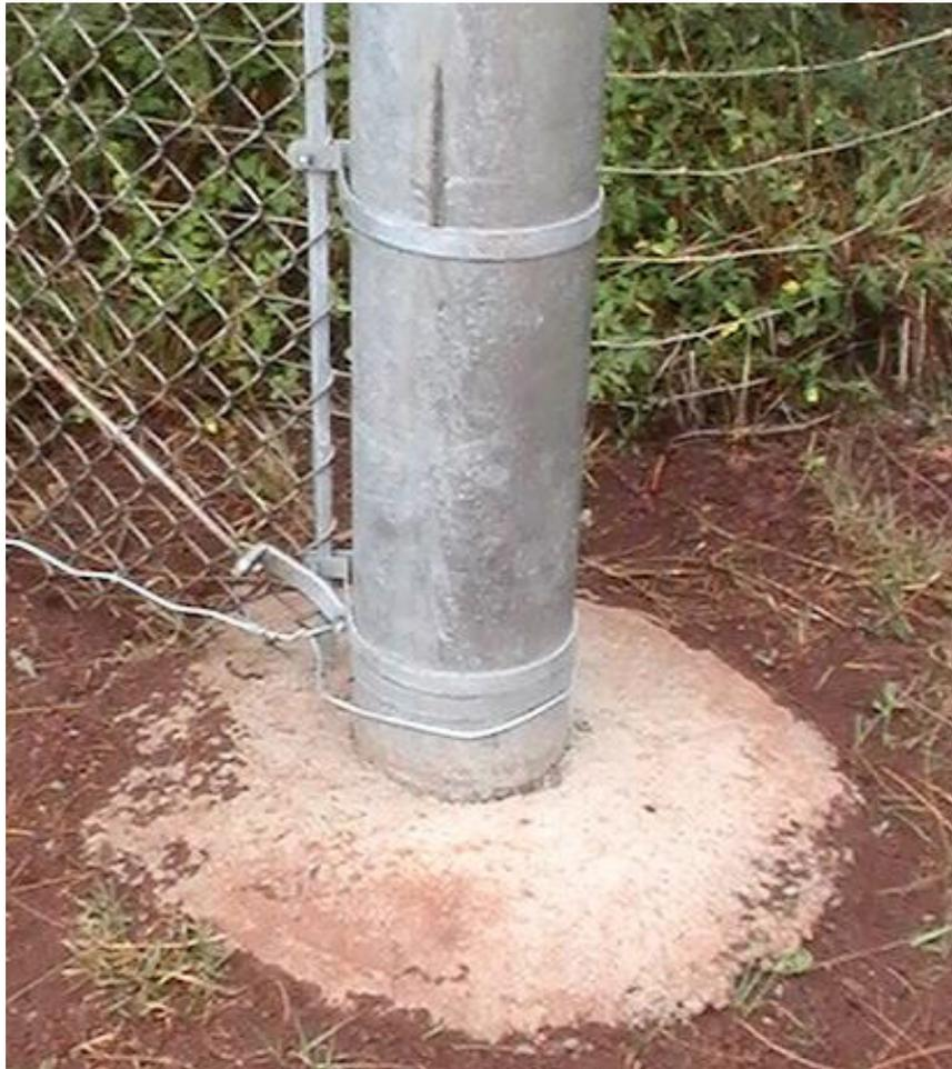
Figure 6. Position-locking hardware for vehicle gates.
