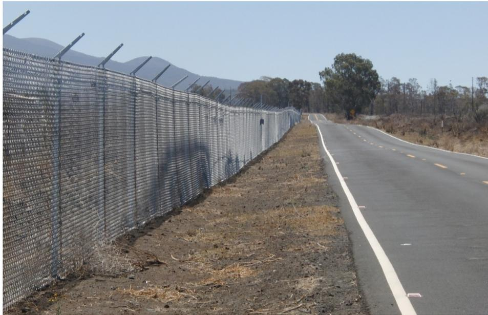
**Figure A3. Fuse-bonded PVC fencing at west BAA perimeter from Old Saddle Road to New Saddle Road (right) and four test sections of control materials (left).**
