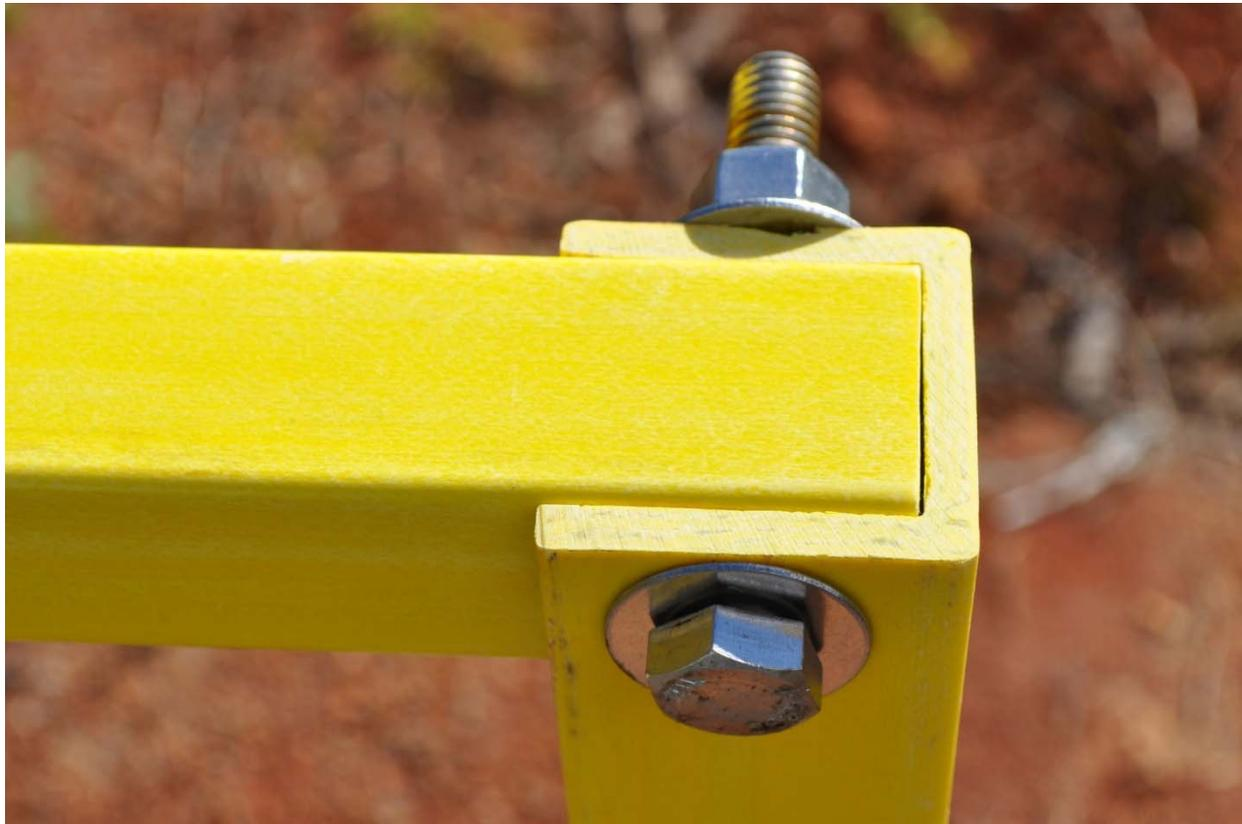
Figure B78. Fabricated FRP Railing
