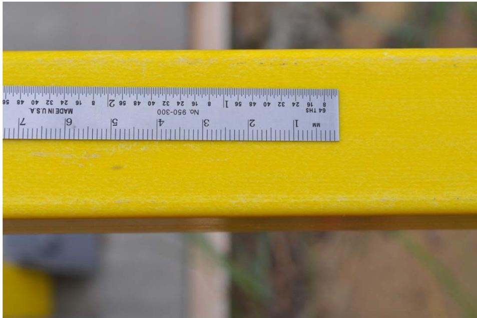
Figure B2. Fabricated FRP Railing
