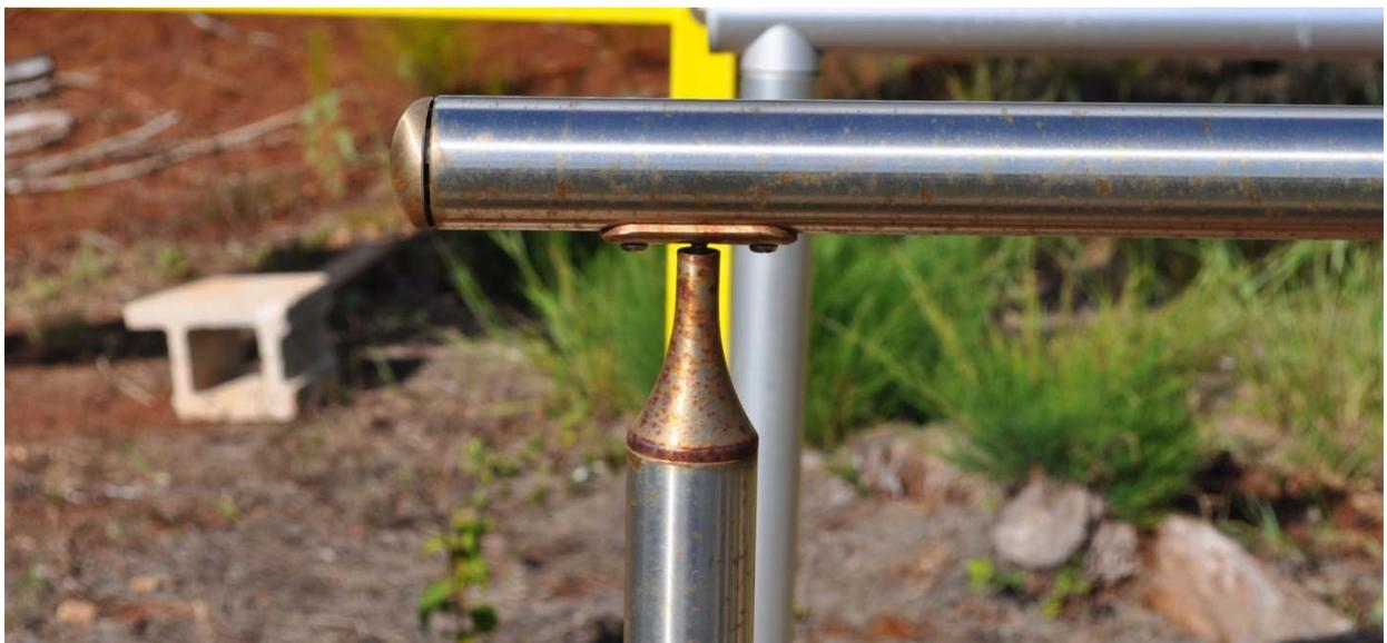
*Figure B82. Stainless Steel T-fittings on fabricated railings*
