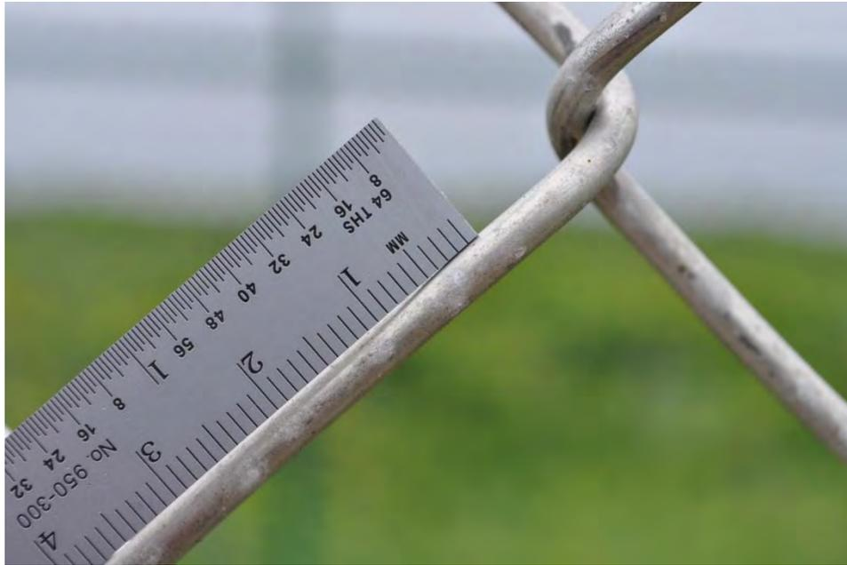
Figure B12. Aluminized Steel Wire Fencing
