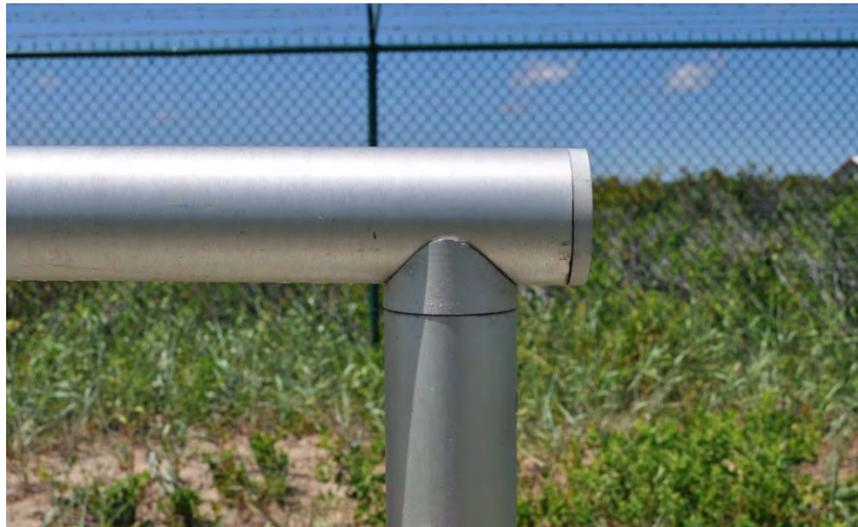
Figure B28. Fabricated Aluminum Railing
