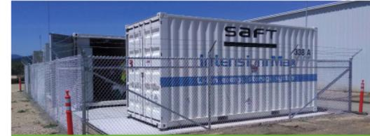
Figure 1. Fort Hunter Liggett installed a lithium-ion battery to help mitigate demand charges and reduce PV curtailment. The battery was purchased with funding from the Army's Energy Resilience & Conservation Investment Program. Photo by Lars Lisele, NREL.
