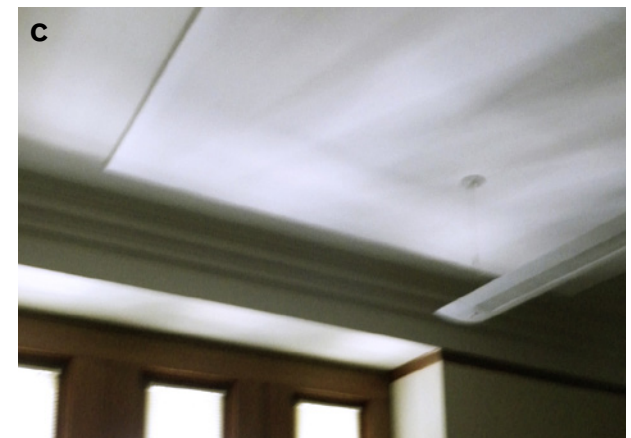
AFTER: Stretched acoustic material applied to ceiling
