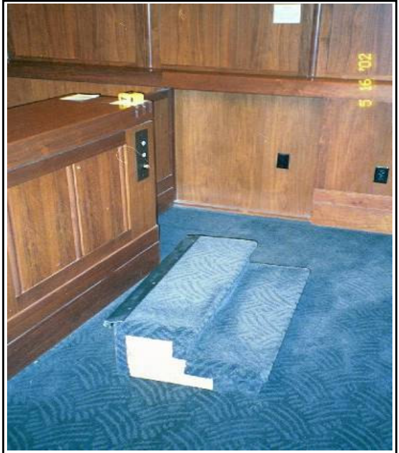
Stair Element (Witness Box)
