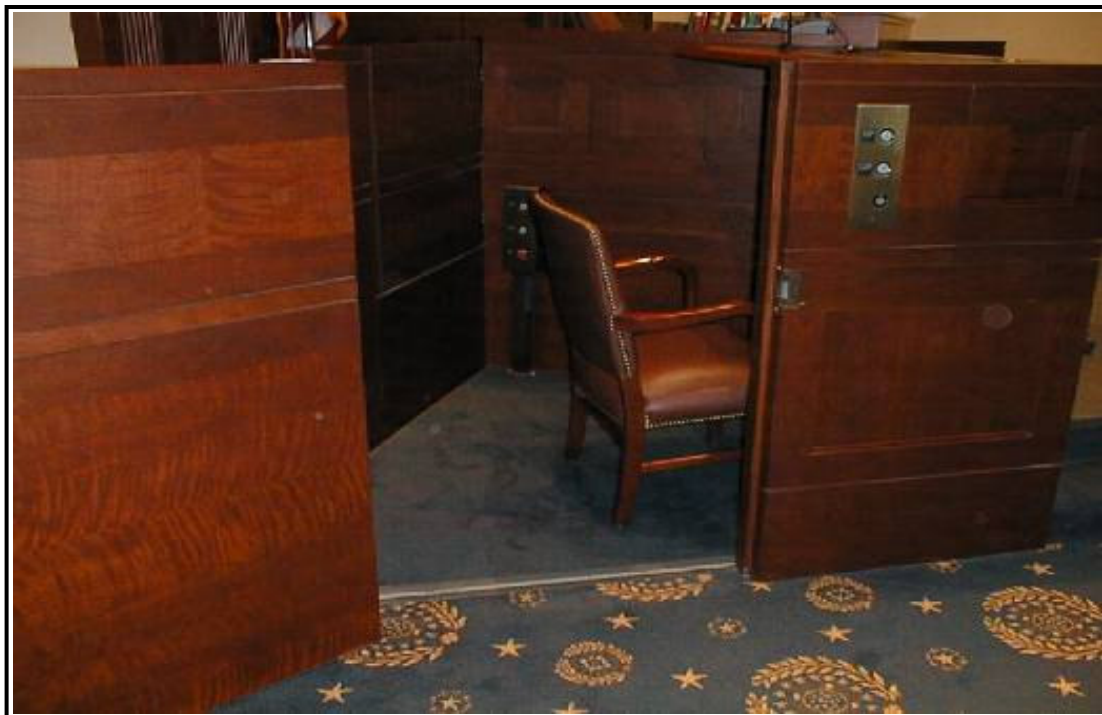
Note: Substantially Differing Heights Of Lift Controls
