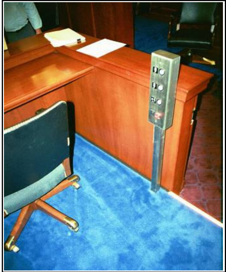
Lift Controls On Platform
