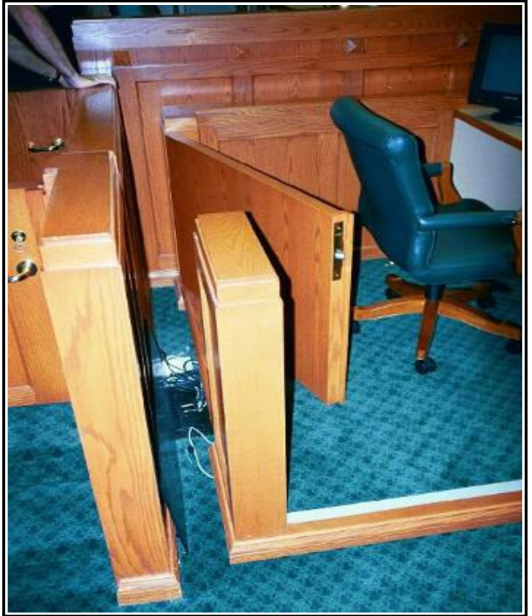
Gap Between Lift Area And Witness Box
