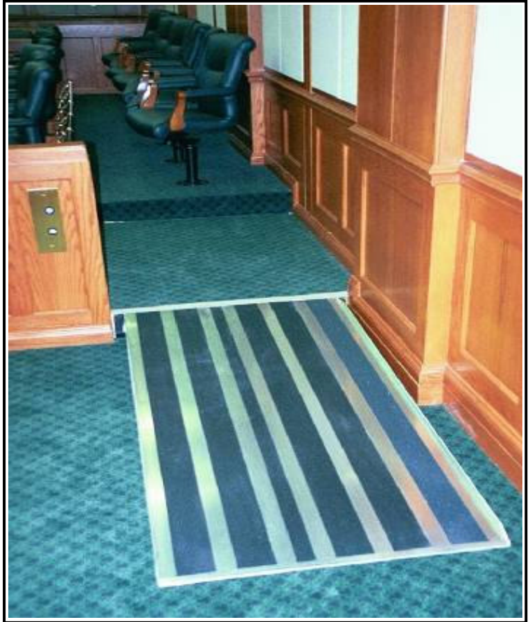
Fully Extended Ramp At Jury Box
