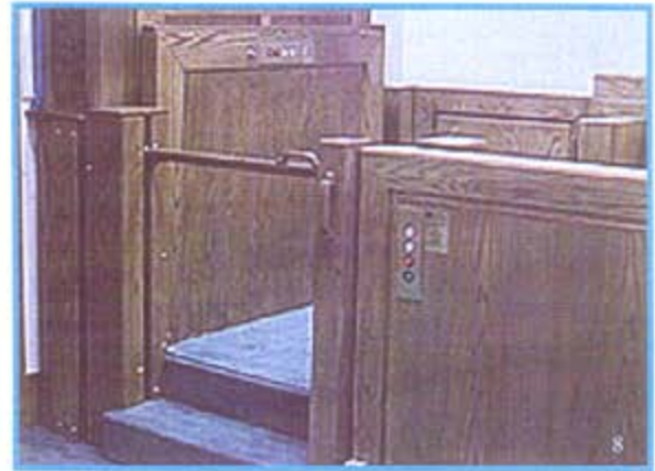
Barrier arm up — ready for platform to lower for access
