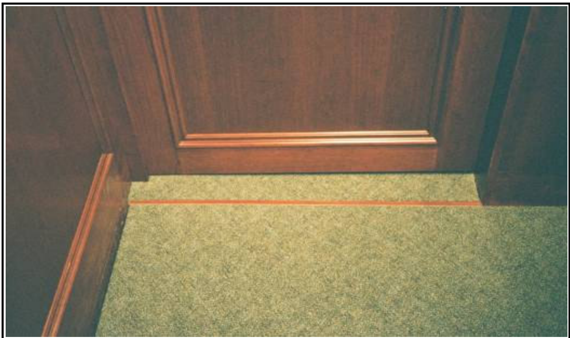
Gate And Floor Joint Within The Witness Box
