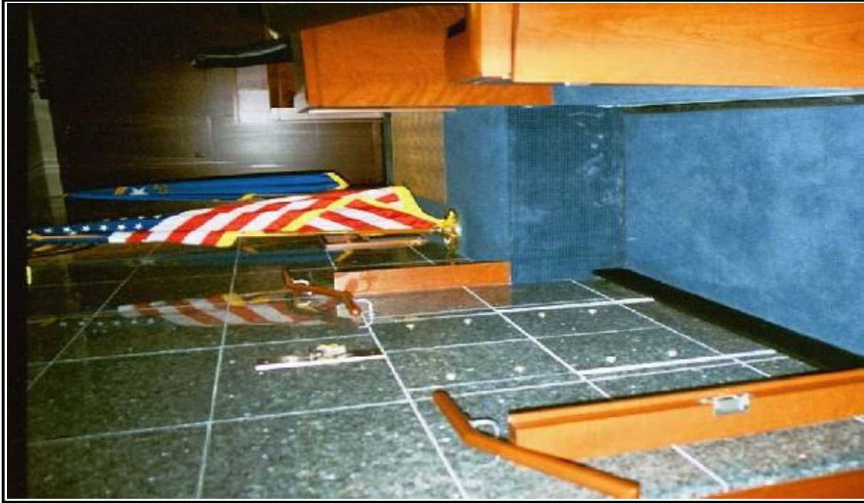
Looking At The Lift Area From Courtroom Well Area
