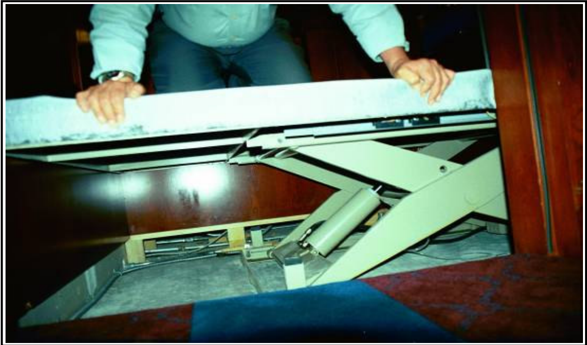
Platform Framing And Scissors Lift Mechanism
