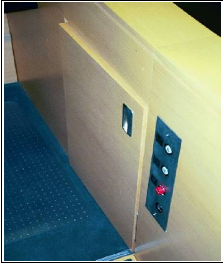
Folding Panels Protruding From Recess
