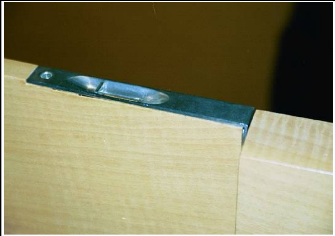
Clamp At Top Of Folding Panels
