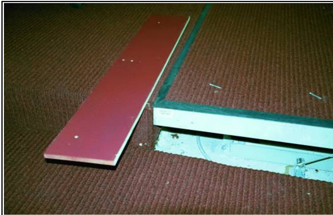
Wood Riser Removed For Service Access
