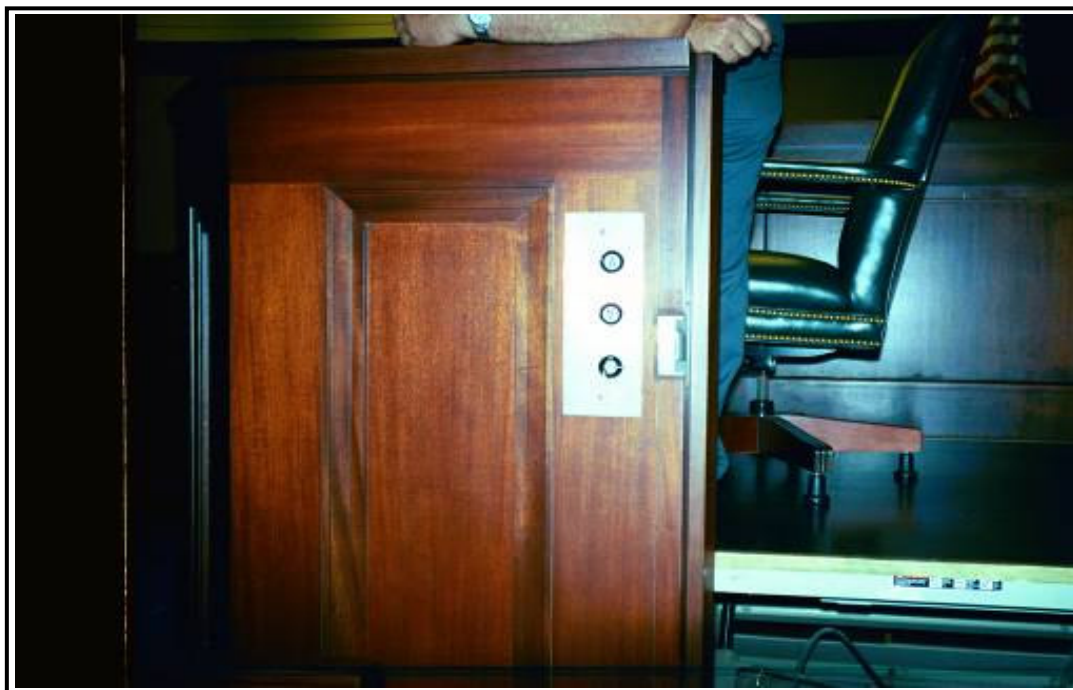
Lift At Witness Box Level / Controls / Exposed Mechanism
