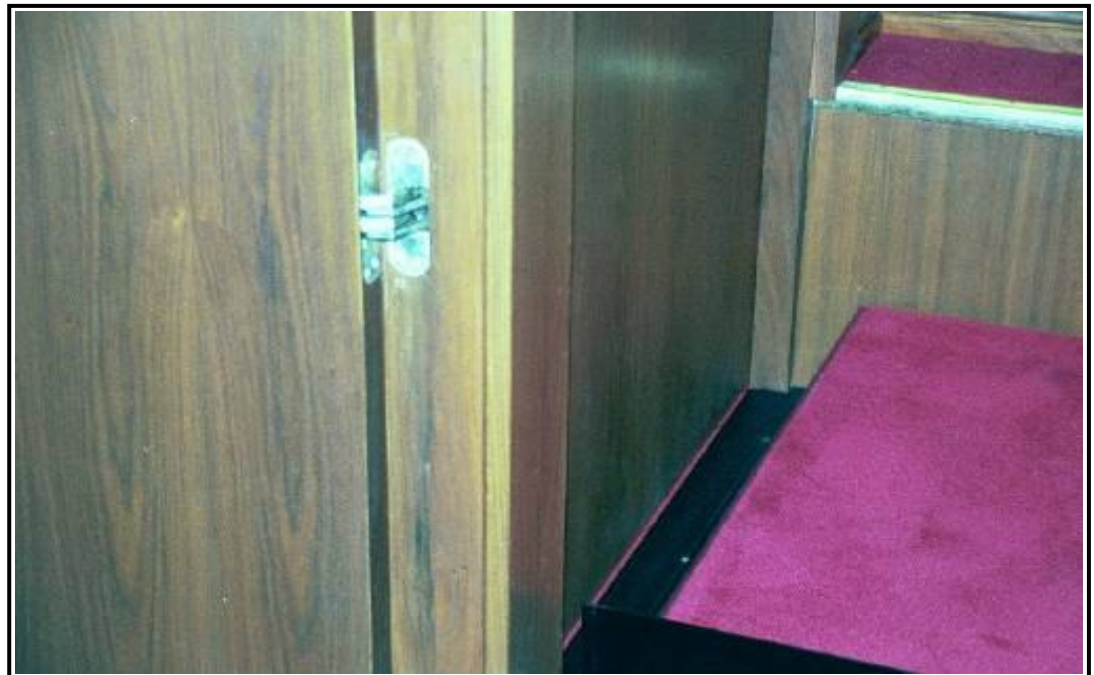
Hinge At Gate Enclosing Lift
