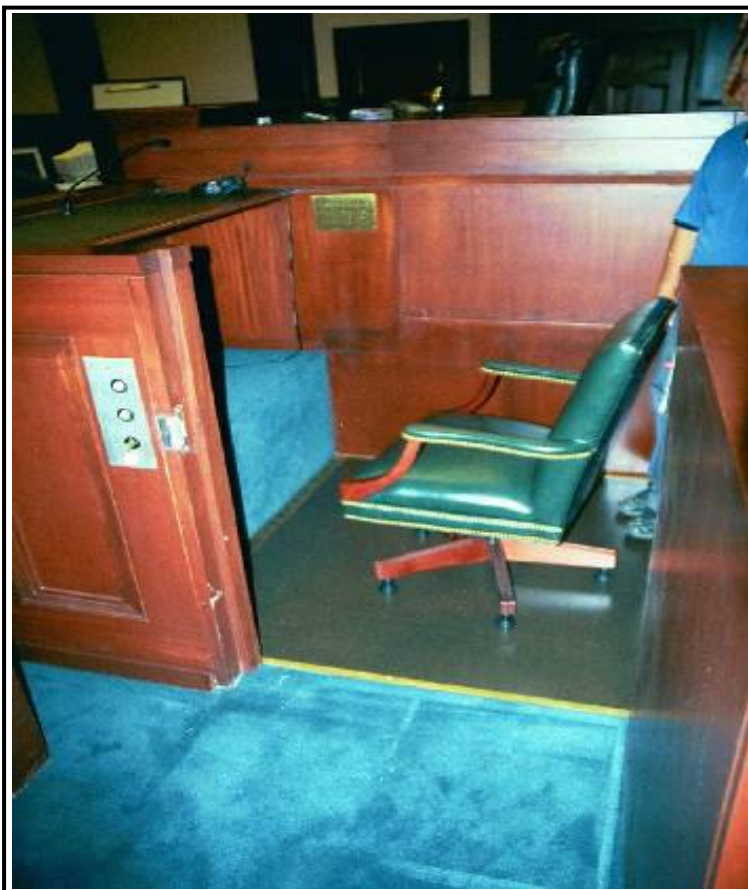
View Into Witness Box - Lift At Lowest Level
