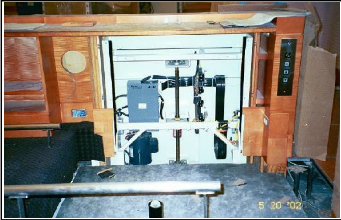
Acme Screw Drive Recessed Into Millwork Enclosure
