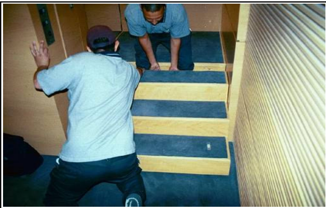
Removal of 3-Step Riser
