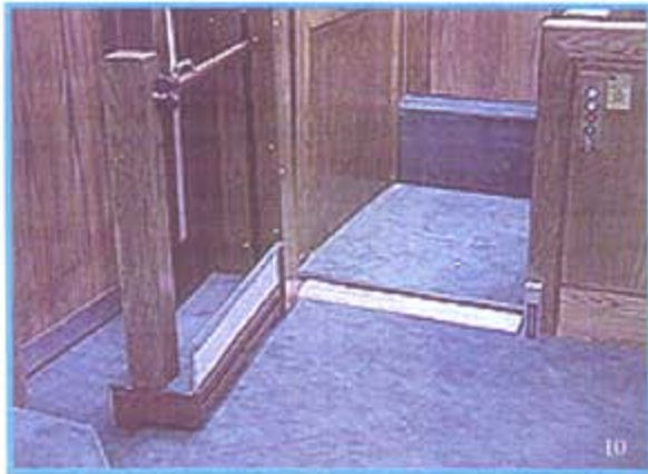
Platform lowered for wheelchair access — gate/step hinged open
