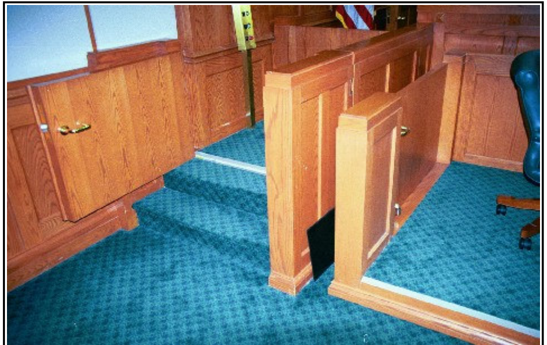
Millwork At Lift And Witness Box
