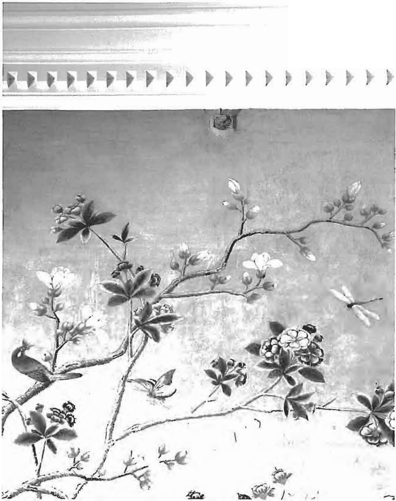
Figure 1. Blair House, the Presidential guest quarters, Washington, DC, has undergone a fire safety retrofit. A sprinkler head is visible below the cornice line.
