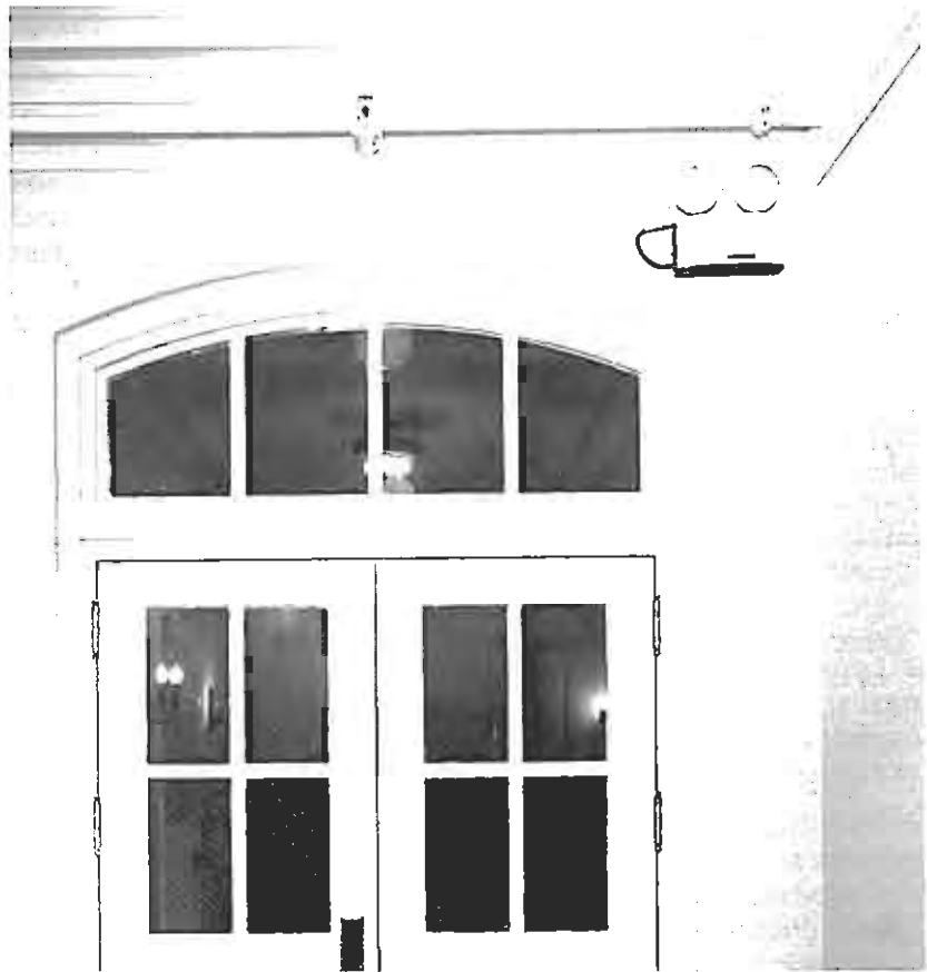
Figures 16 and 17 (below left and immediately below). In the Jackson Place sitting room at Blair House, sprinkler heads have been thoughtfully positioned relative to ceiling moldings.
