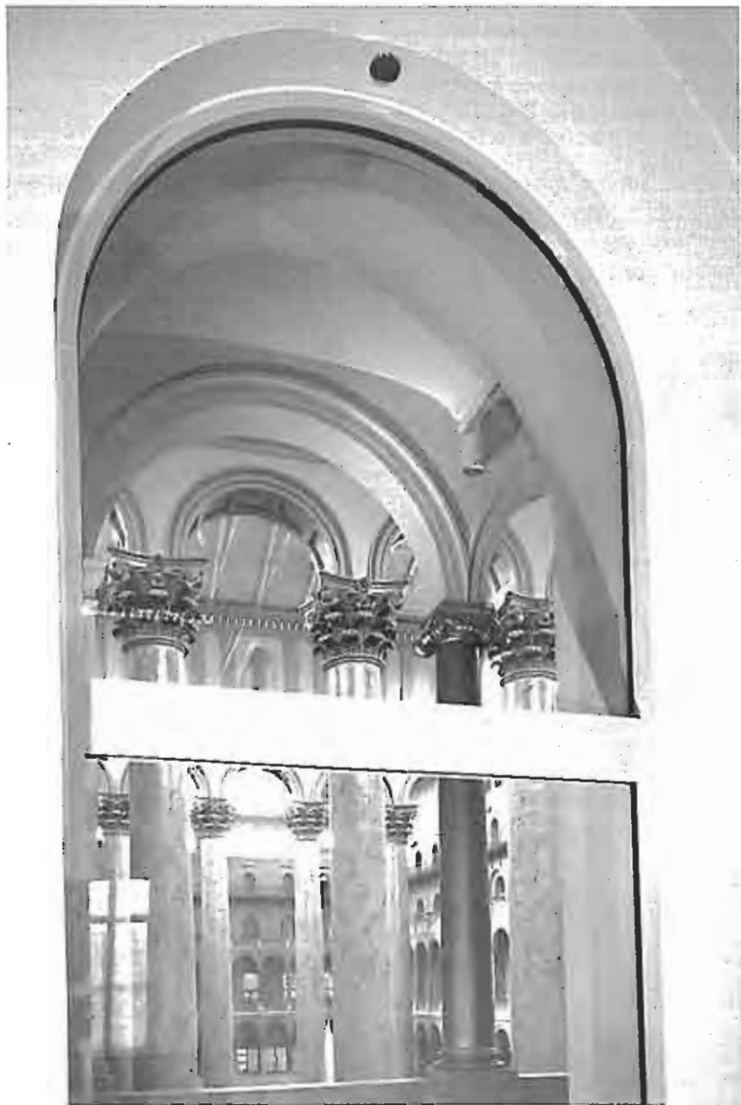
Figure 11 (left). The resulting sprinkler head is quite unobtrusive: it is the circular brass plate atop the window arch. The window looks out over the central atrium.
