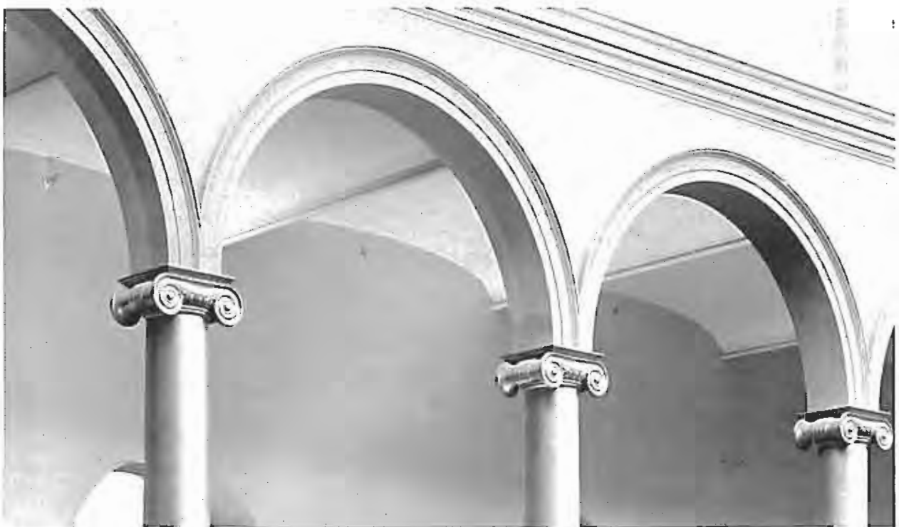
Figure 9. Sprinkler heads are tucked under the vaulted ceiling arches at the National Building Museum, Washington, DC.
