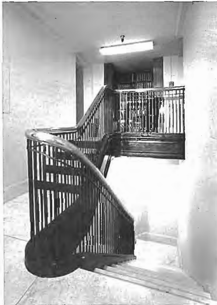
Figure 8 (below). The new landing of this same stair.
