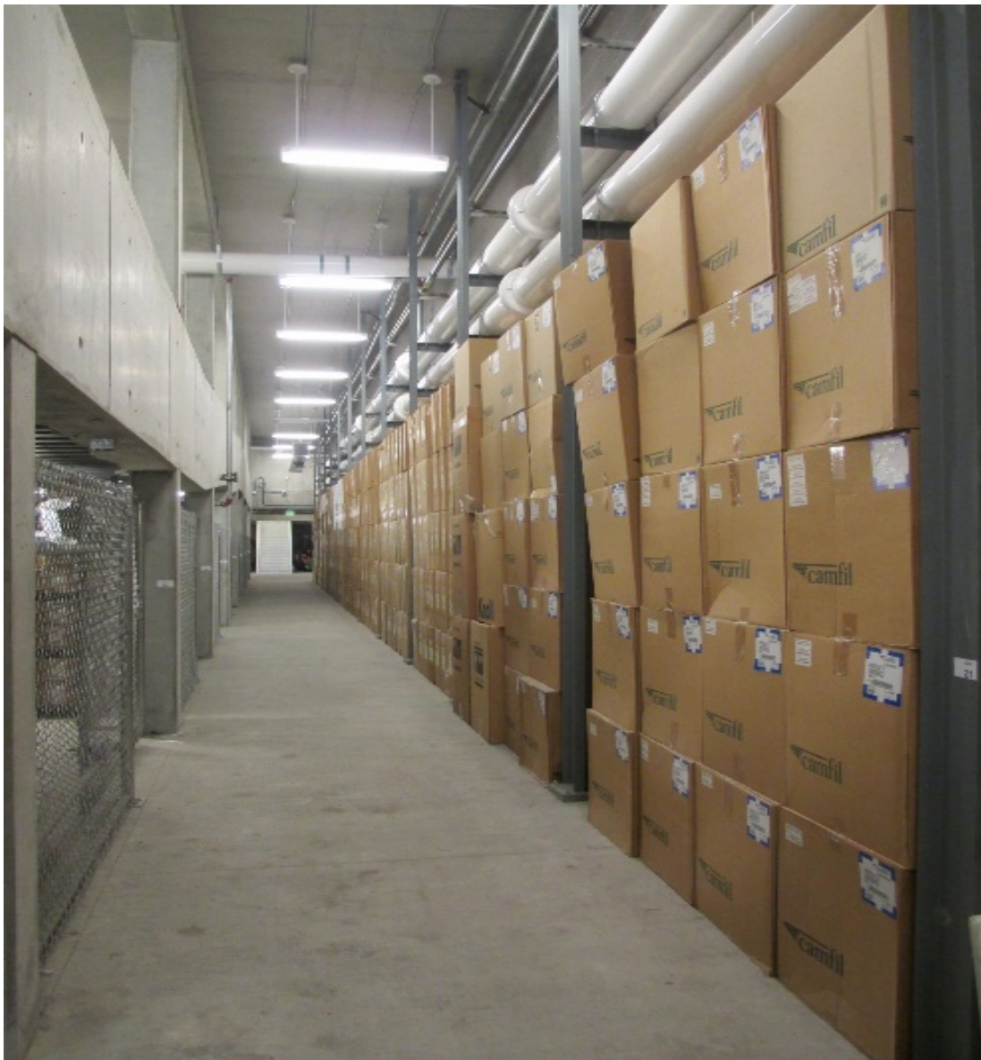
The many neatly stacked boxes should have been anticipated in storage design, to avoid storing in the corridor.
