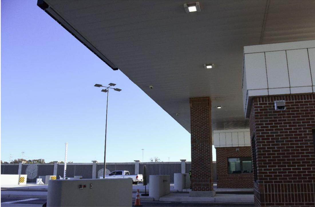
Figure 13 - Canopy luminaires do not provide any indirect light on underside of canopy
