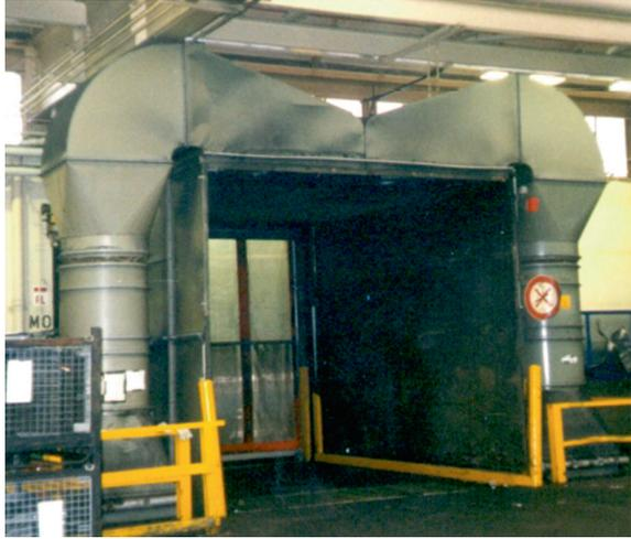
**Fig. 2.18** Scheme of combined air curtain with a lobby: (1) heated air curtain; (2) outdoor air curtain, (3) lobby [2]
