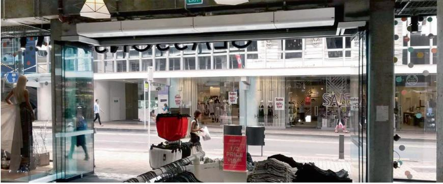
**Fig. 2.13** Example of mixing air curtain with a vertical air supply use at a shopping mall (Frico, Sweden)
