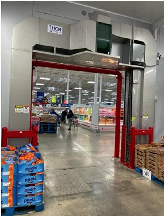
The lobby length is selected such that the supply air is not forced outside. To shorten the length of the lobby, the air can be supplied with an incomplete fan jet from a specially constructed outlet. The air curtain can include medium pressure axial fans mounted on top of air distribution ducts.
