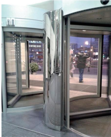
**Fig. 5.10** Revolving door with a concave profile single-sided MAC
