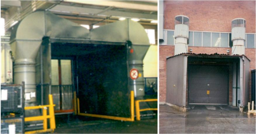
**Fig. 2.1** Examples of protected apertures of industrial facilities equipped with air curtains: **a** Machining shop of Ford Werke, Koeln-Neil, Germany; **b** Scania Cabin Plant in Oskarshamn, Sweden. *Source* A. Zhivov [2, 3]
