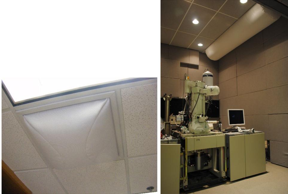
Figure 6-6. Textile air dispersion diffusers can eliminate the probability of condensation by using porous fabric diffusing the air (courtesy of Duct Sox Co.).
