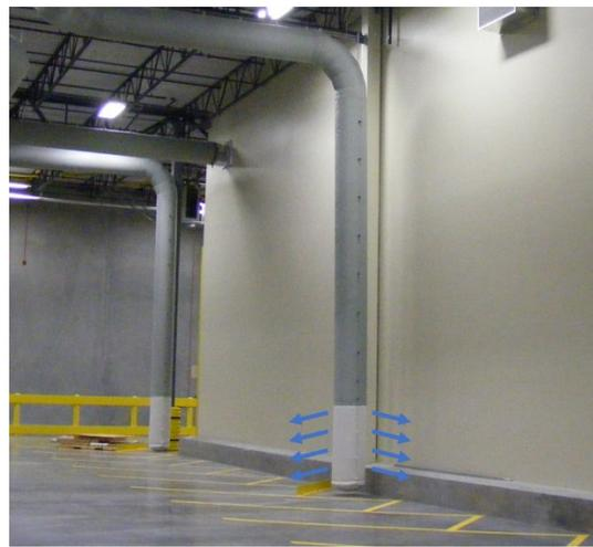
Figure 3-8. Textile Air Dispersion system dispersing displacement supply air at very low velocities using fabric porosity (courtesy of DuctSox Co.).
