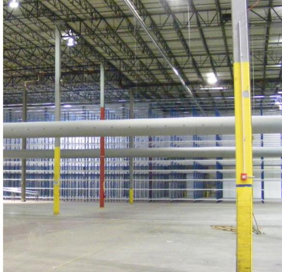
**Figure 3-11. Textile Air Dispersion system mounted at less than half of ceiling height and with air dispersion orifices for active displacement ventilation (Courtesy of DuctSox Co.).**
