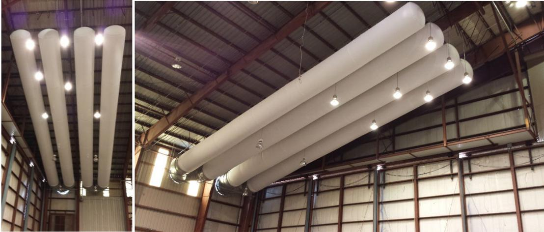
**Figure 2-3. A bank of textile air dispersion systems using only the fabric porosity to create an air shower over a painting area.**
