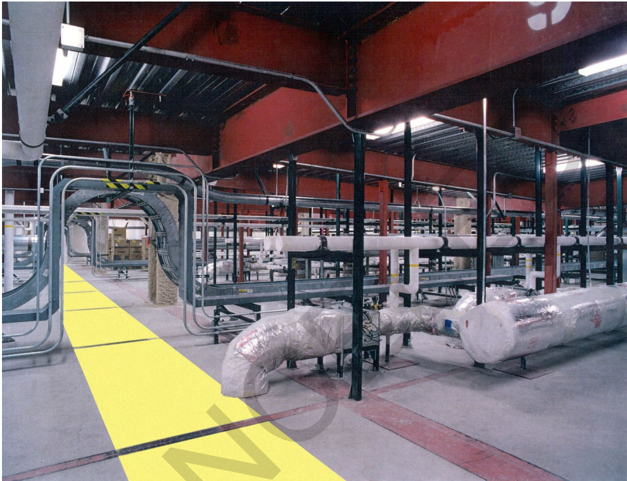
Figure E-3 Interstitial Access-Egress (Typical)
