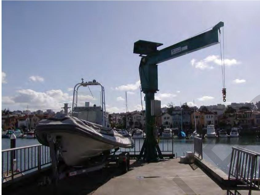
Figure 8-2, Small Craft Crane Access (Jib-boom)
