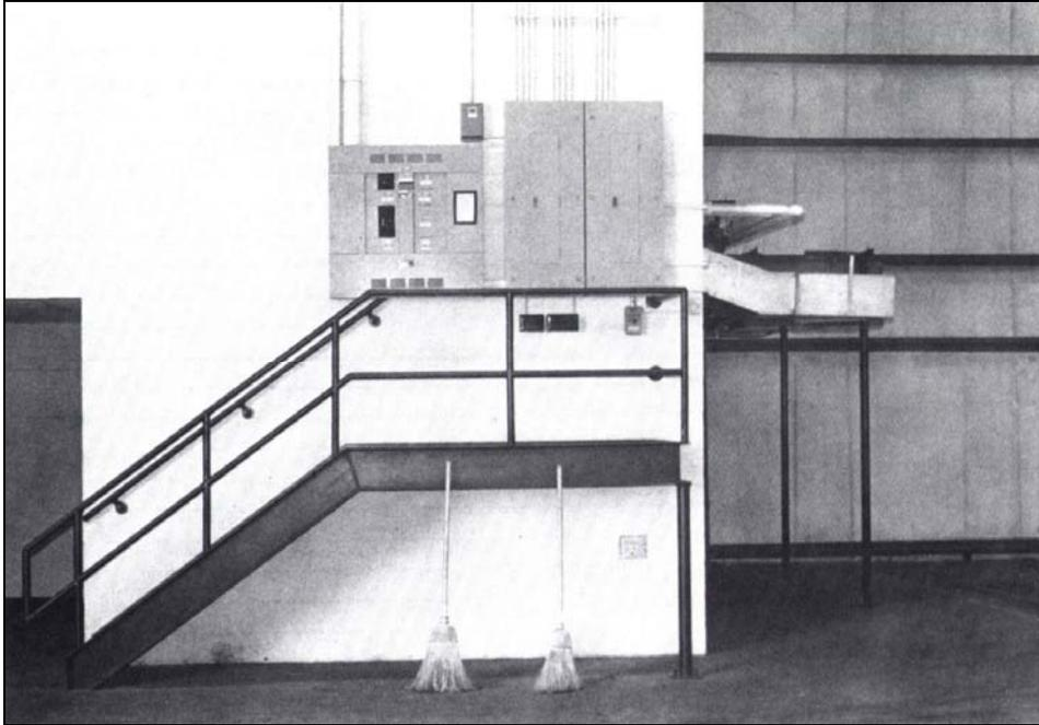
**Figure 6-5. Electrical utilities elevated for protection against flooding**
