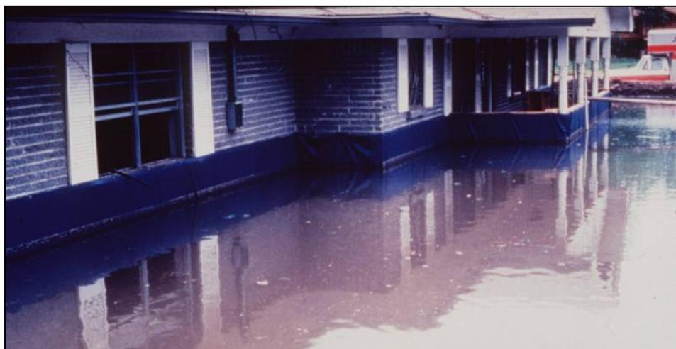
**Figure 7-2. Photograph of membrane providing flood protection**
