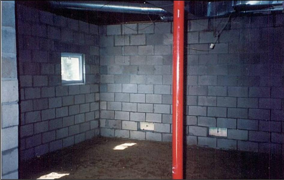
**Figure 8-4. New foundation with vents**
