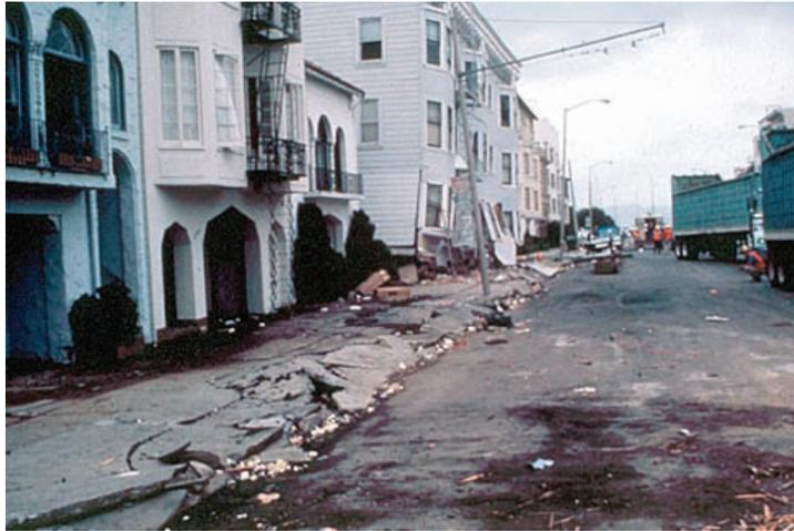
Sand boils and flows on the surface can displace and damage structures and utilities. Lateral liquefaction flows will result in subsidence, loss of foundation integrity, disruption of underground utilities and damage to structures resting on the soil surface, including roadways and utility structures. Liquefaction susceptibility and potential should be identified in the site geotechnical investigation, as explained in Section 3.3.3.
