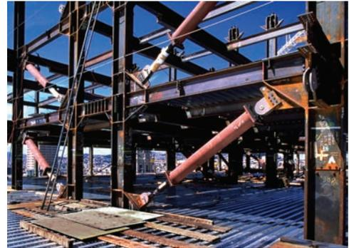
3. **Unbonded steel braces** with the brace providing stable tension-compression behavior, a significant improvement over the conventional braced frame.
