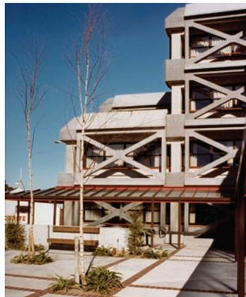
Figure 5-42: Exposed cross-bracing examples.
