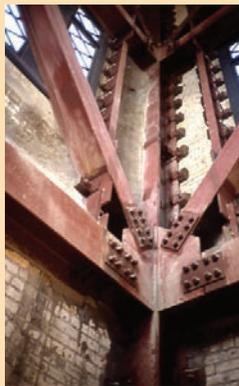
Figure C: Steel space frame inserted within tower
