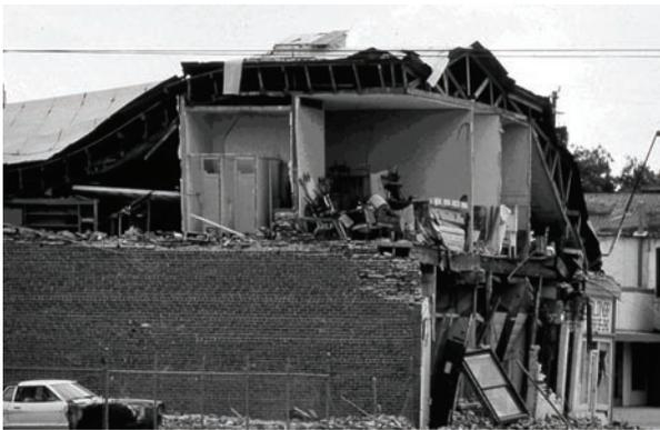
Figure 9-4: Nonstructural partition walls prevented the total collapse of this unreinforced masonry structure in the 1983 Coalinga earthquake.
