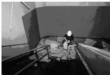
Figure 9-6: Difficulty in exiting due to debris strewn across exit stairs can be an indirect threat to life, as can be seen in this photo following the Loma Prieta earthquake in 1989.
