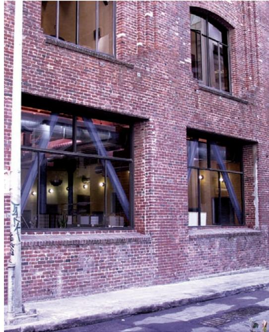
Figure 8-13: Examples of the many configurations of steel braced frames used in commercial retrofit in San Francisco.
