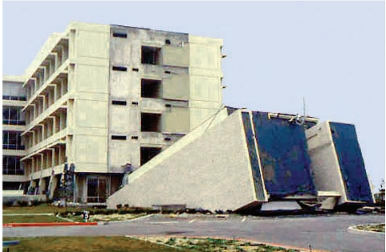
Figure 8-2: Olive View Hospital. A brand new facility that was damaged beyond repair in the 1971 San Fernando earthquake due to a shaking intensity that exceeded what was expected at the site and a design that, although technically complying with code at the time, contained several structural characteristics now considered major deficiencies. The lateral system contained nonductile concrete frames, discontinuous shear walls, and a significant weak story.
