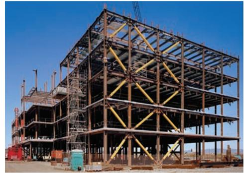
4. **Coupled 3-part systems with moment frames, links, and shear walls** to provide a progressive resistance system in which the resistance progresses from the most rigid system to the more ductile-flexible system.
