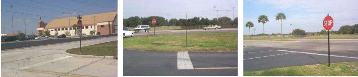
Figure D-1 Example of Stop Lines
